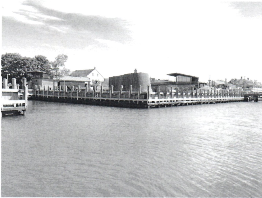
Figure 2-6: View of Bulkhead looking Northeast
