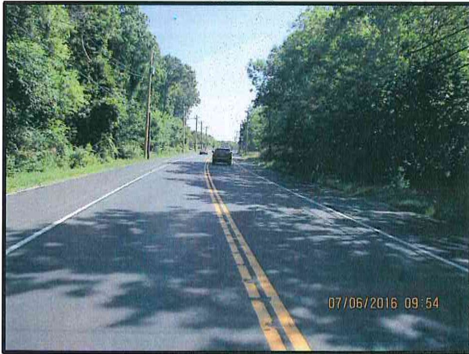
Photo 3 – View looking northeast on Route 25.
