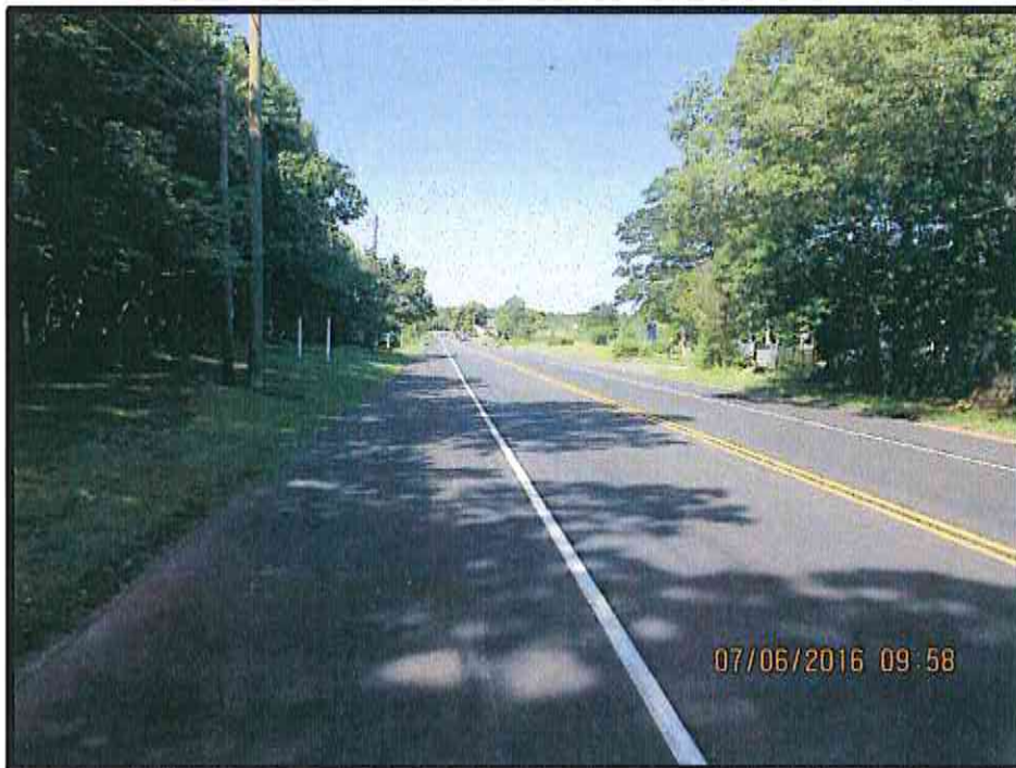
Photo 10 – View looking west-southwest on Route 25; adjacent to New York State DOT yard.
