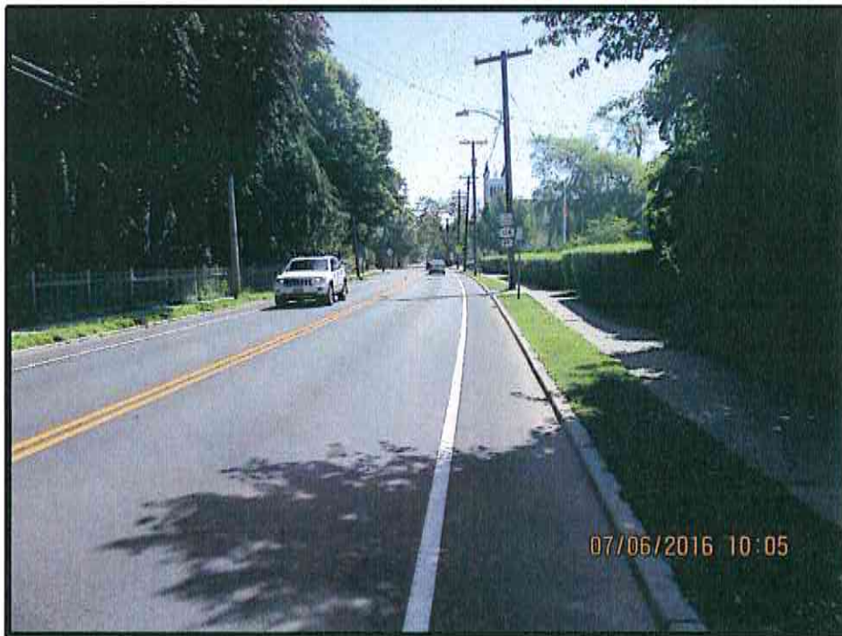
Photo 22 – View looking east on Route 25.
