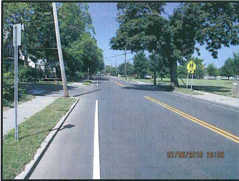
Photo 21 – View looking west on Route 25.
