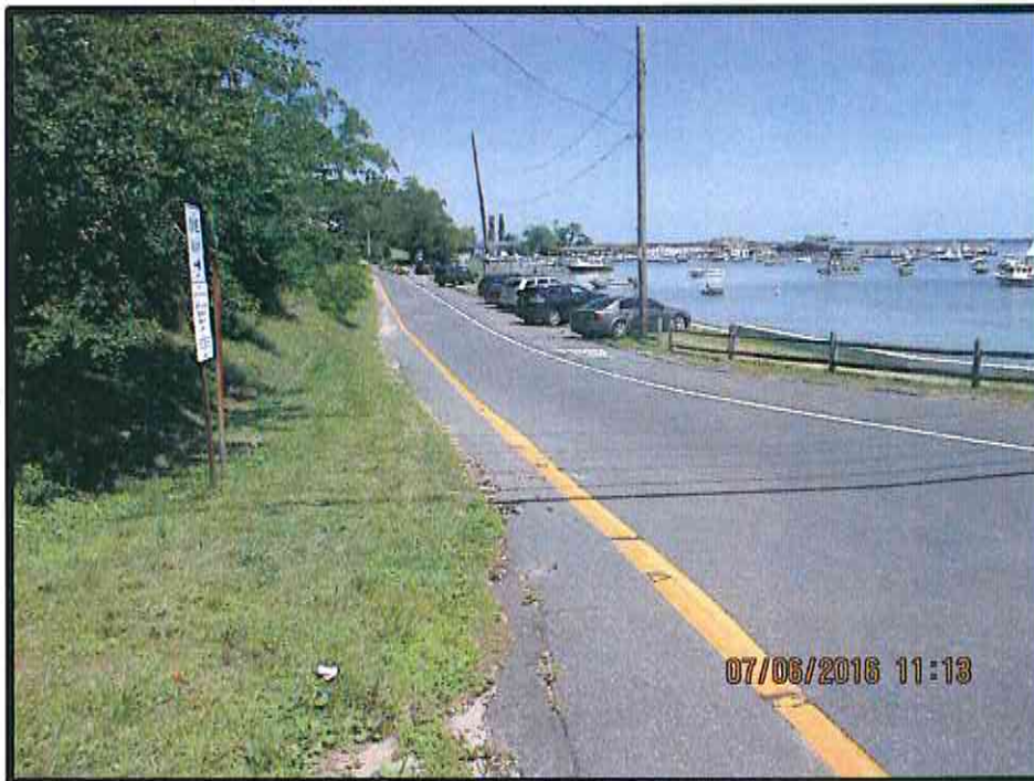
Photo 52 – View looking north on Cedar Avenue.
