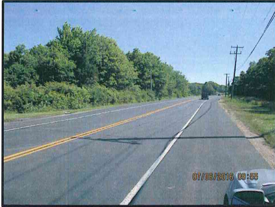
Photo 5 – View looking northeast on Route 25.
