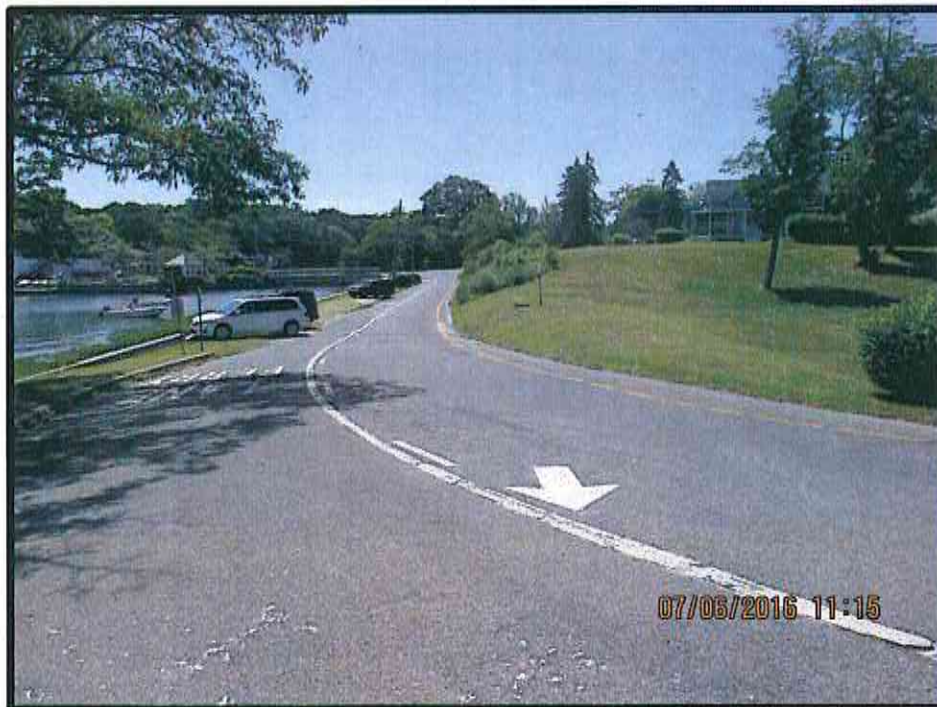
Photo 50 – View looking south on Cedar Avenue.
