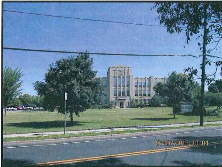
Photo 19 – View looking north on Route 25; adjacent to Greenport High School.
