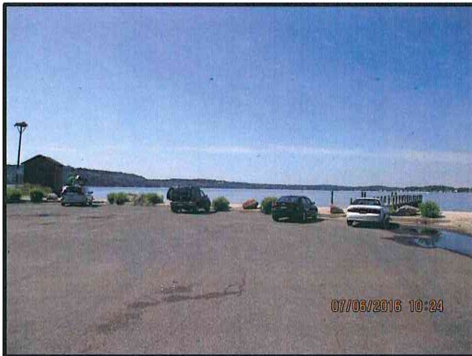
Photo 40 – View looking south towards Shelter Island Sound North; are is the proposed location of drill pit.
