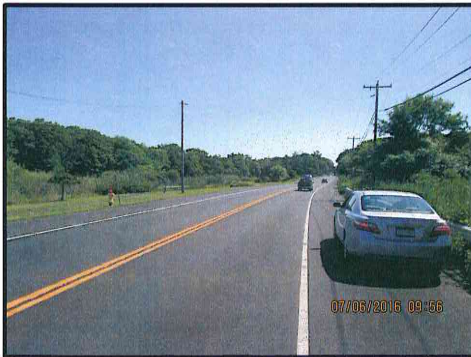
Photo 8 – View looking east on Route 25.
