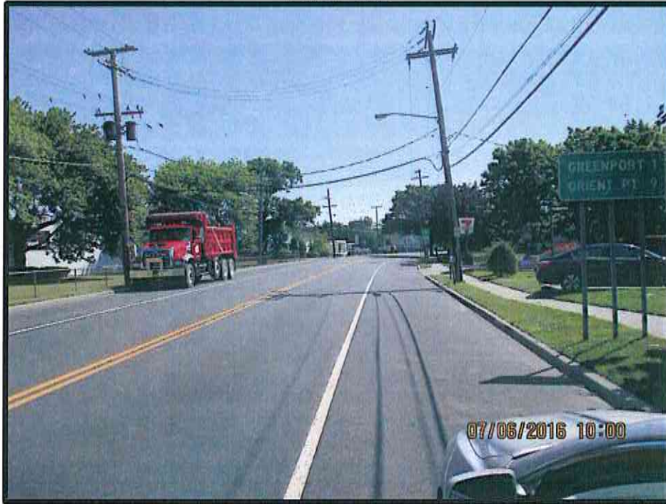
Photo 15 – View looking east-northeast on Route 25.
