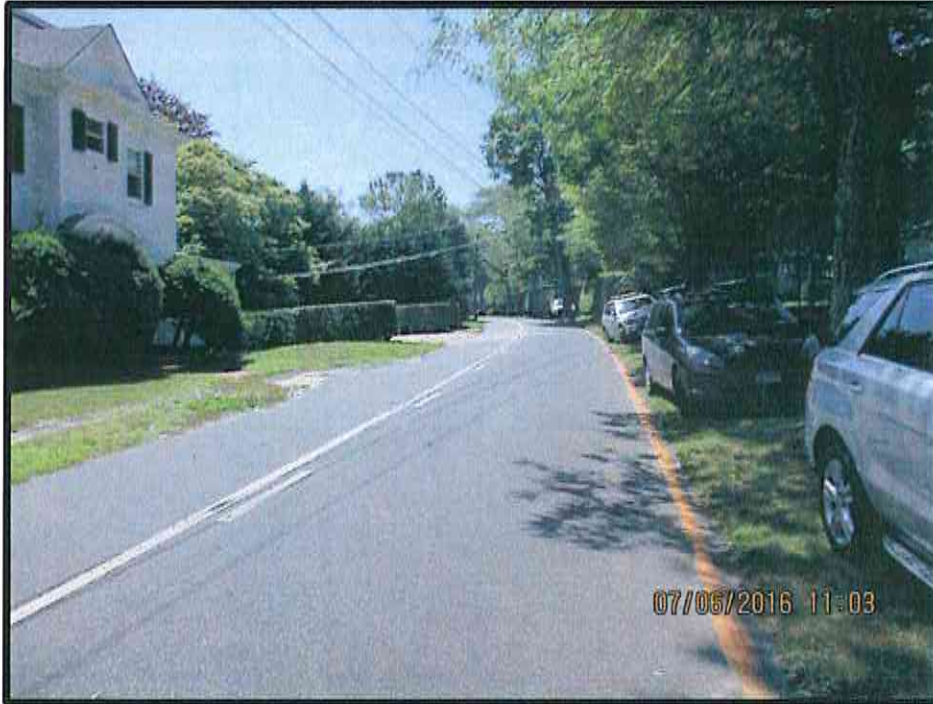
Photo 47 – View looking south on Clinton Avenue; adjacent to village tennis courts.
