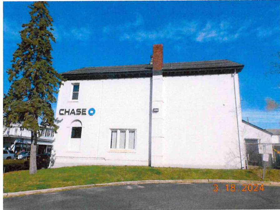
PHOTO NO. 03 SOUTH ELEVATION
