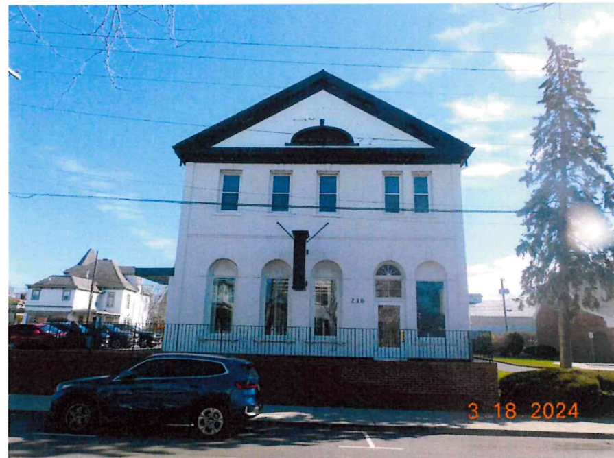
PHOTO NO. 04 WEST ELEVATION
