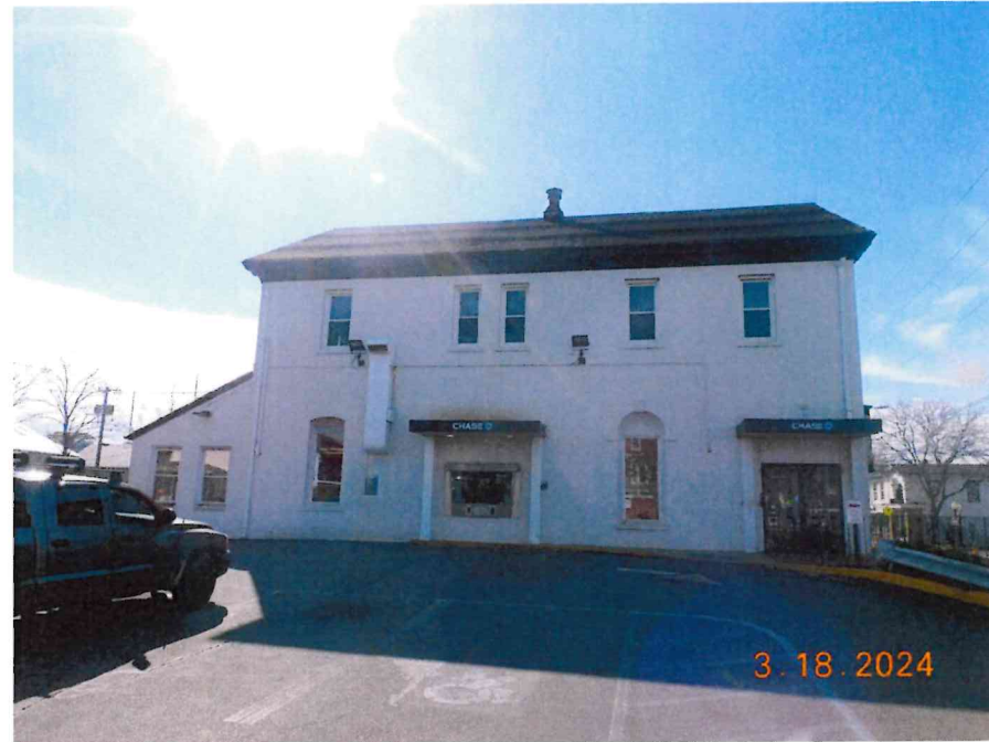
PHOTO NO. 01 NORTH ELEVATION
