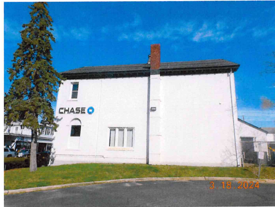
PHOTO NO. 03 SOUTH ELEVATION
