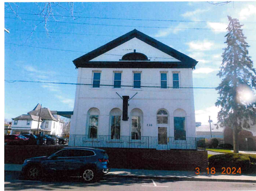
PHOTO NO. 04 WEST ELEVATION
