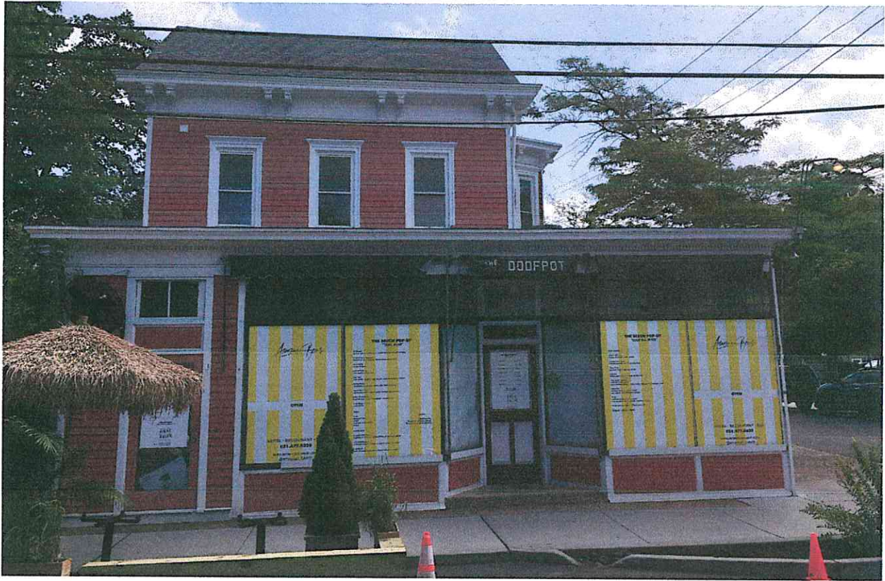
WEST ELEVATION (MAIN STREET) - REPAIR AND REPLACE EXISTING TRANSOM WINDOWS AND AWNING IN KIND
