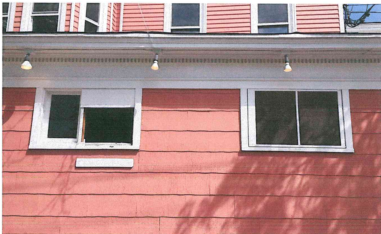
SOUTH ELEVATION (BAY AVENUE) - REPLACING FIRST FLOOR WINDOW SASHES IN KIND
