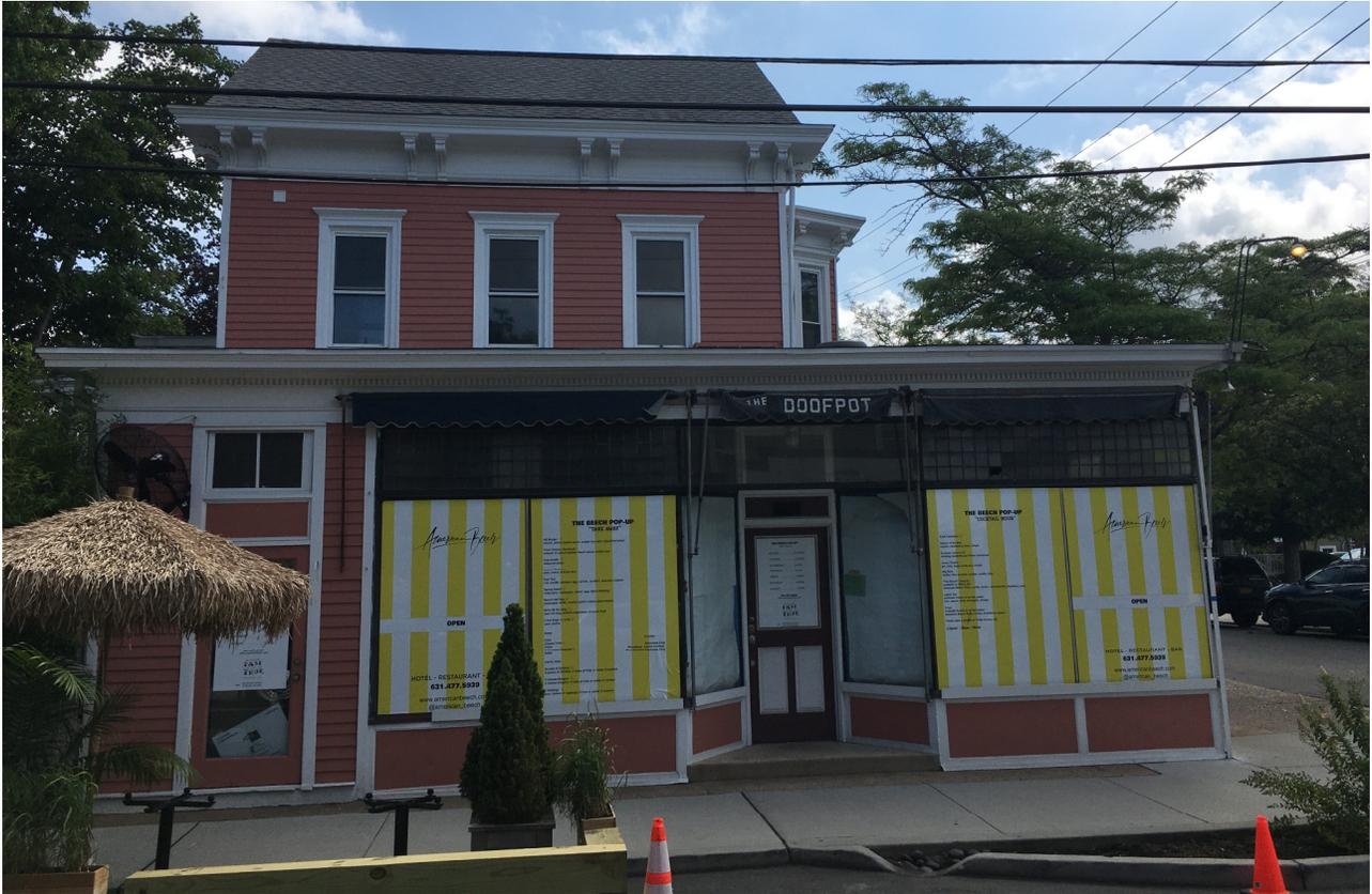
WEST ELEVATION (MAIN STREET) - REPAIR AND REPLACE EXISTING TRANSOM WINDOWS AND AWNING IN KIND
