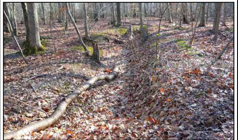
A series of man-made drainage ditches were constructed which provide a low-cost storm water drainage function, draining the waters that enter Silver Lake. Over time the drainage ditches have filled in with tree limbs and other natural debris which have decreased their effectiveness. The Village is considering community participation projects with groups like the Boy Scouts to help clear these areas.
